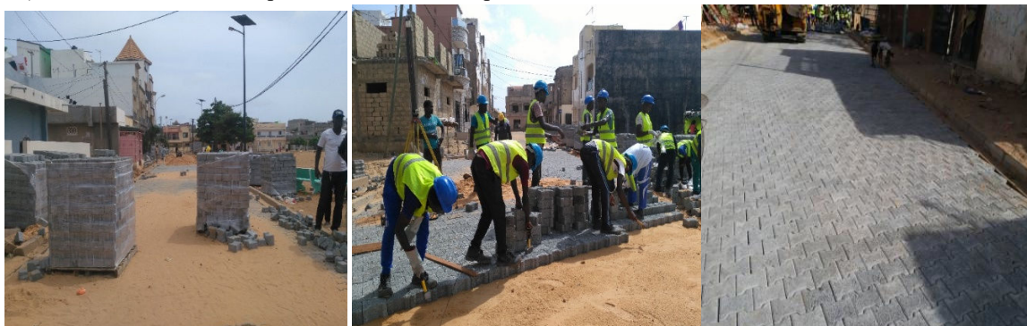
Figure 12: Photographs pavement of roads
