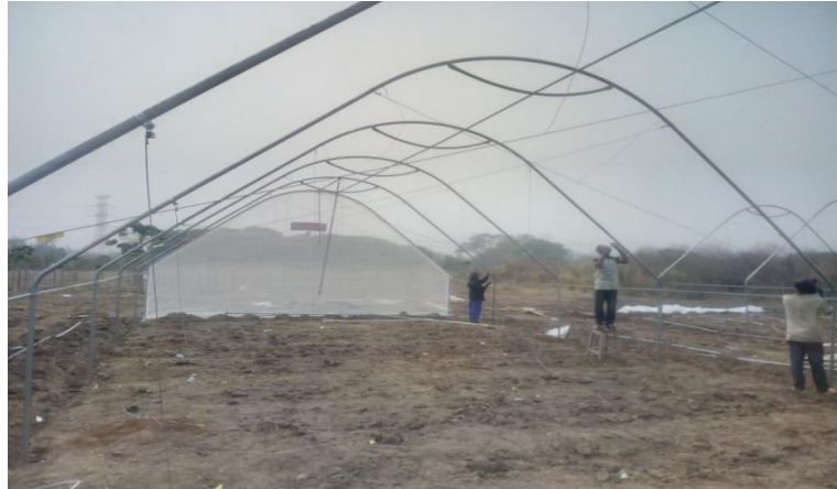
Plate1. A Quonset greenhouse under construction
