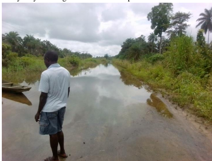
Figure 1: Road leading to Federal University Otuoke completely submerge under water
