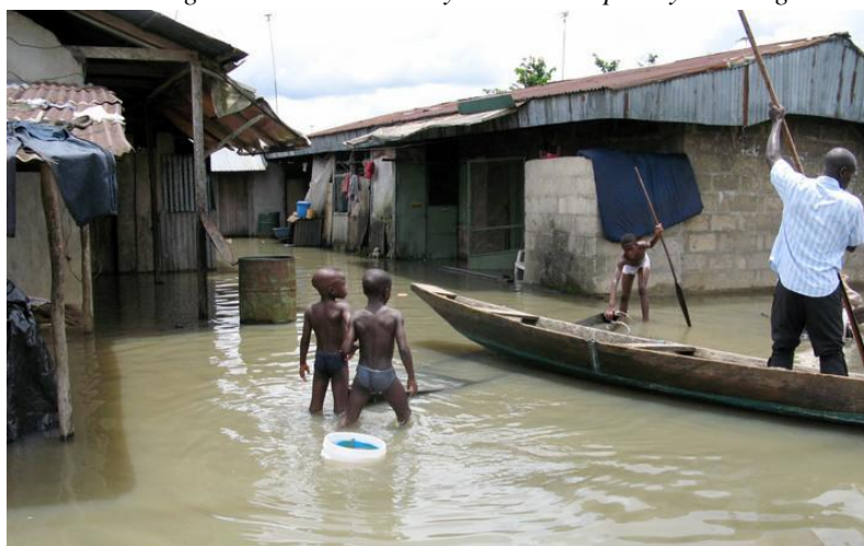
Figure 2: Flooded Residential building accessed by boat
