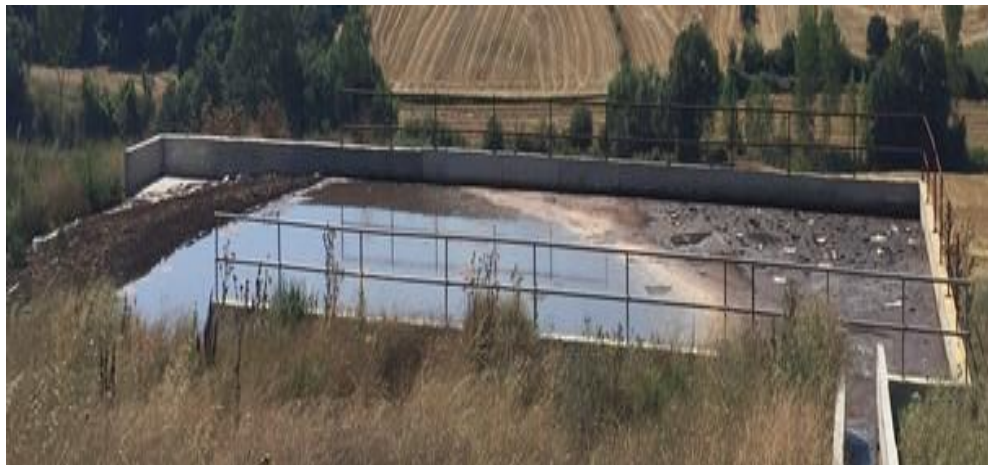
Figure 5: General view of the animal waste warehouse
