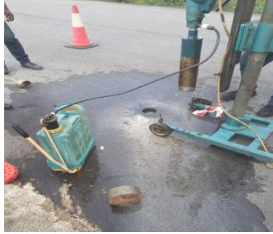
Plate 2.9: Asphalt cored hole
