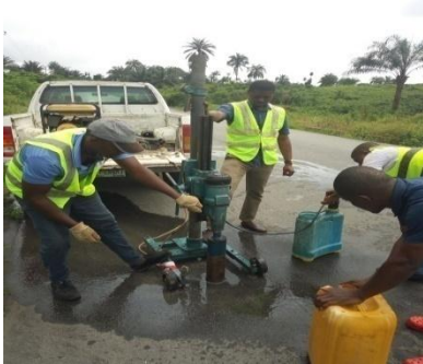
Plate 2.8: During asphalt coring
