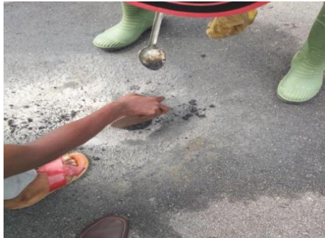
Plate 2.11: Replacement of cored hole with fresh asphalt
