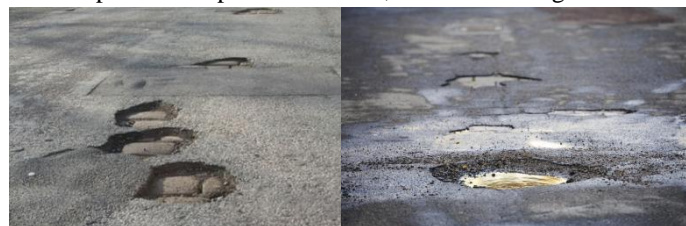
Figure 2: Pavement pothole example reference diagram
