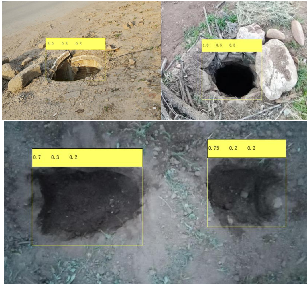
Figure 11: Screenshot of the results of the pothole detection ahead
