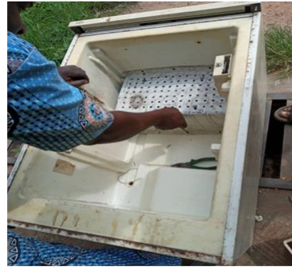
Plate 5: Installation of the Evaporator
