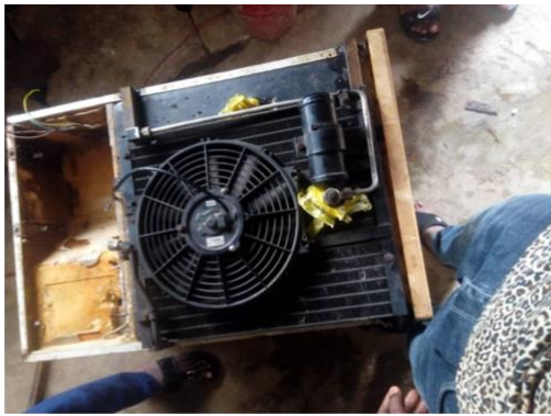
Plate 4: installation of the Condenser to position
