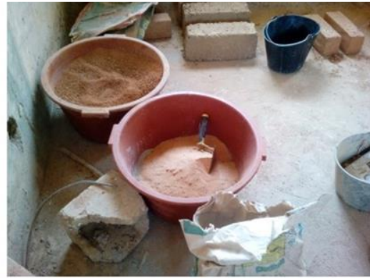
Sieved laterite, sand and cement
