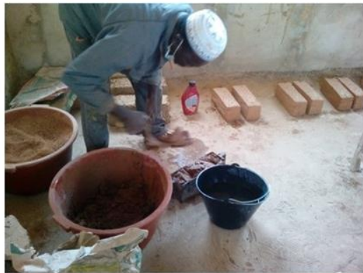
Production of bricks in the artisanal mould
