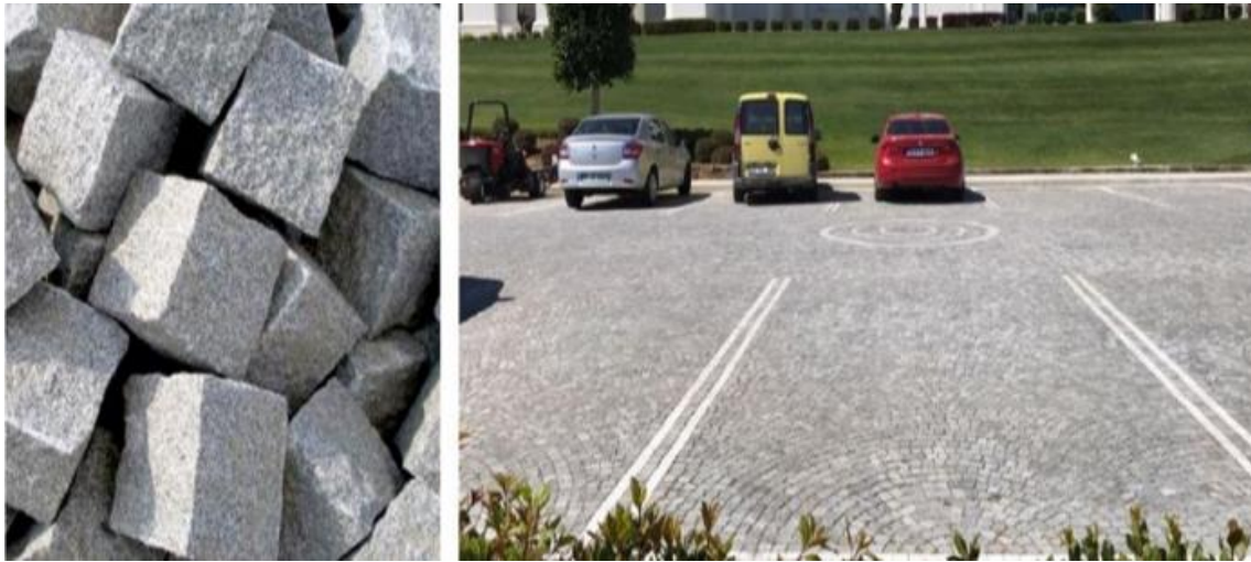
Figure 8: A car parking paved with cube granite-basalt material [10]
