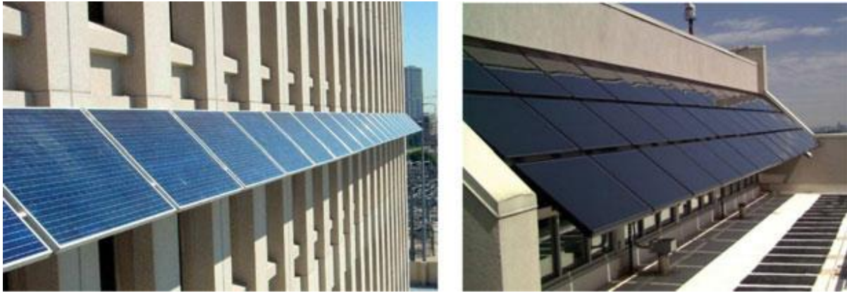
Figure 2: Typical applications of PV shading on buildings [6]
