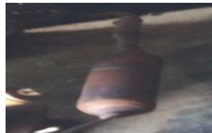
Figure 8: Expansion valve
