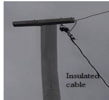
Figure 3: Use insulated cable
