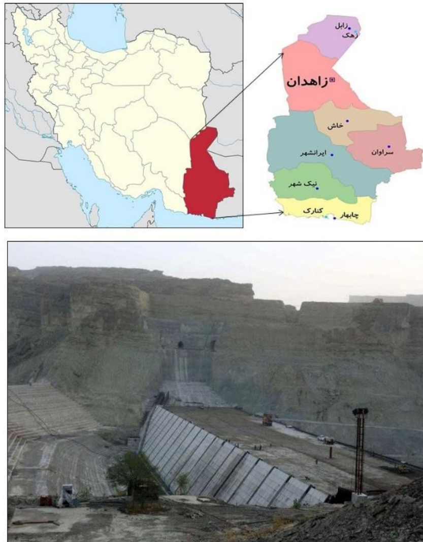
Figure 1: Locating the Kahir Reservoir Dam
