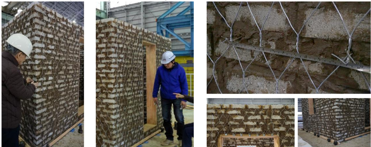
Figure 9: Construction of mud mortar stone masonry houses wrapped with gabion wire mesh.
