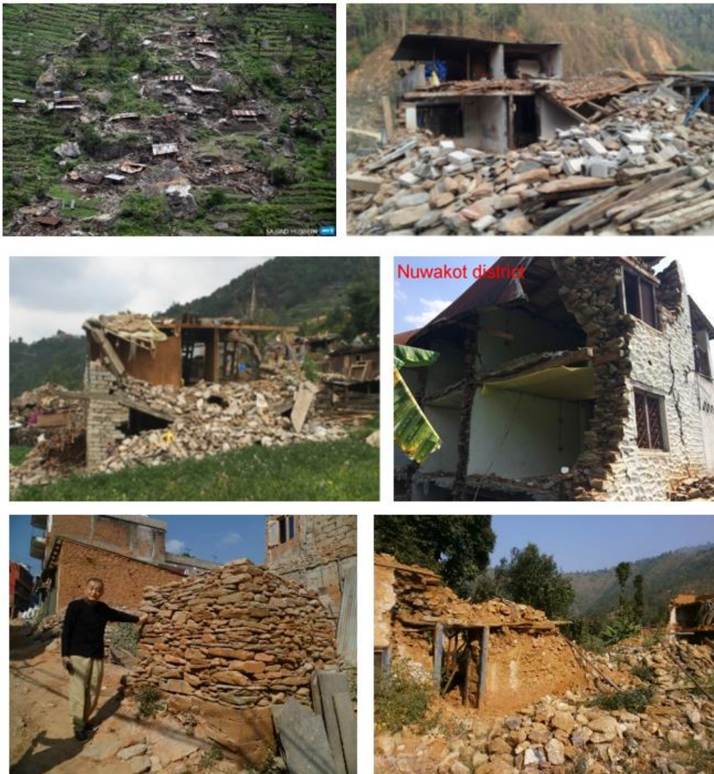
Figure 1: Mud mortar stone masonry houses collapsed due to April 25, 2015 earthquake
