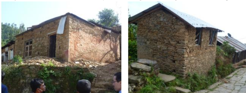
Figure 2: Mud mortar stone masonry houses without horizontal bands
