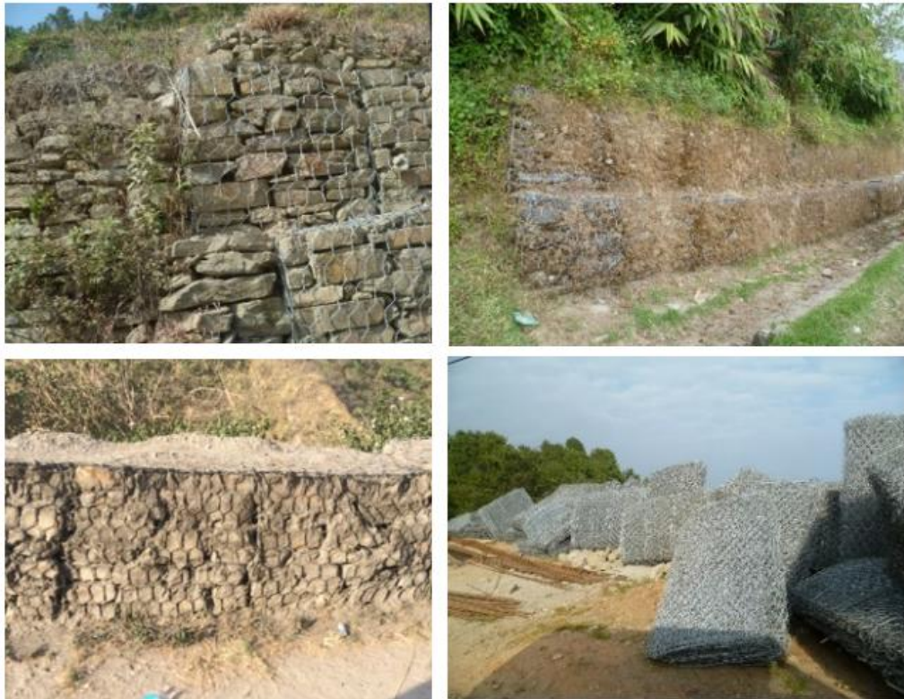
Figure 3: Gabion is used as retaining walls
