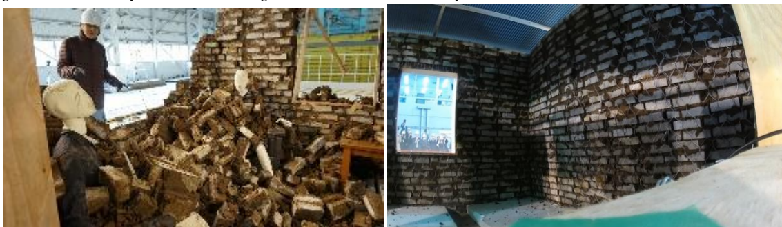
Model A: West and East walls collapsed due to out-of-plane loading; large cracks from window openings in North and South walls
