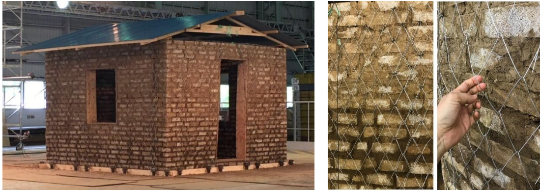
Figure 10: Model B, mud mortar stone masonry strengthened by wrapping 2mm commercial type gabion wire mesh on both sides of the walls, constructed at the end of May 2019
