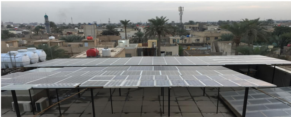
Figure 2: Panels of Solar-powered PV
