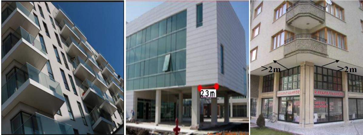
Figure 1: Overhang types: (a) Balcony, (b and c) closed one-sided and two-sided overhangs
