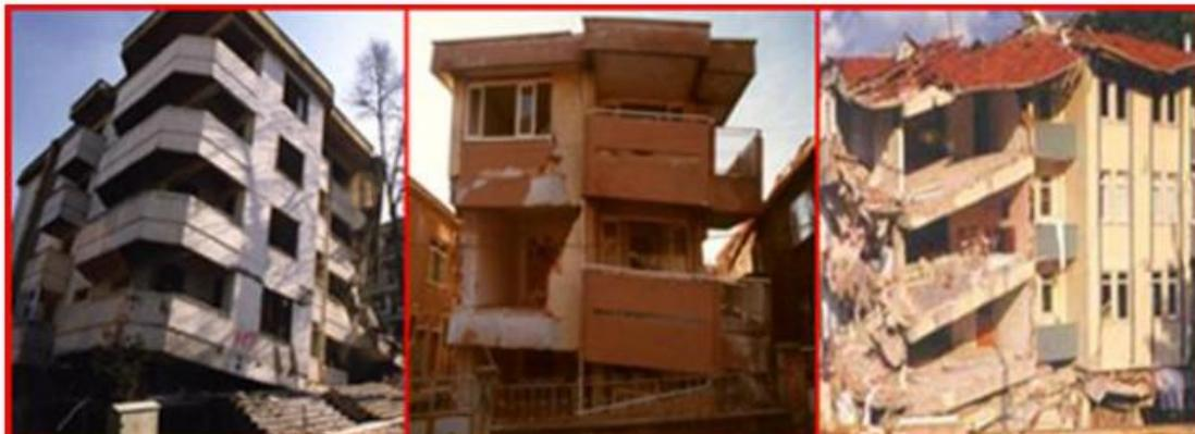
Figure 2: Failure due to overhang
