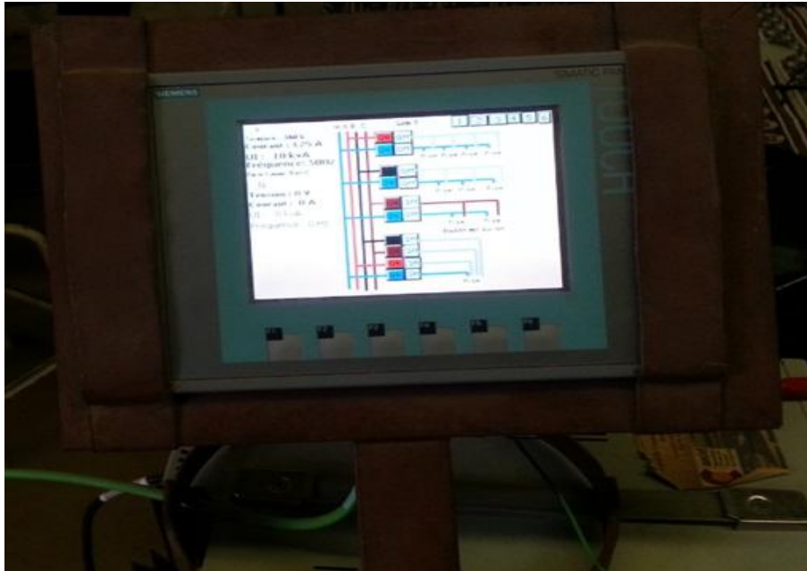
Figure 12: Figure of the SCADA test in the HMI panel of the Research Room
