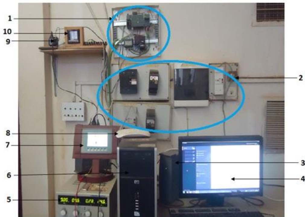
Figure 5: Photo of SCADA control-command
