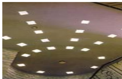
Skylight in the roof
