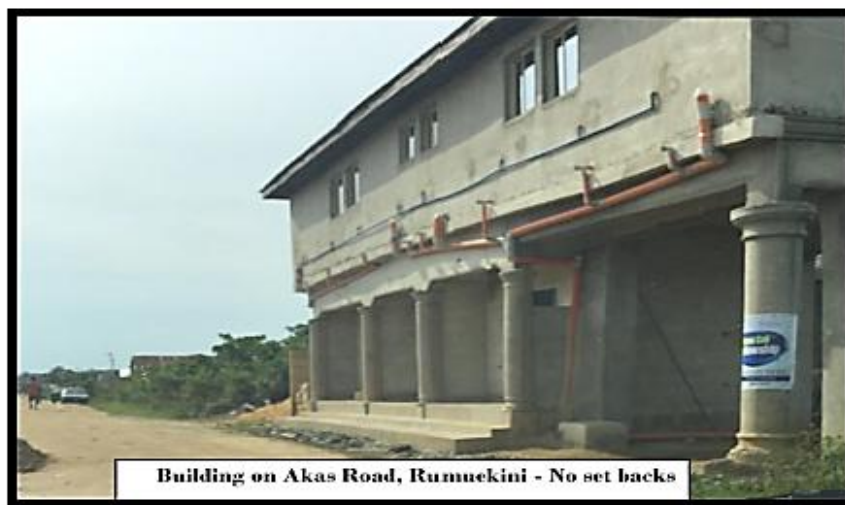
Plate 1: Building Constructed without Setbacks at Rumuekini
