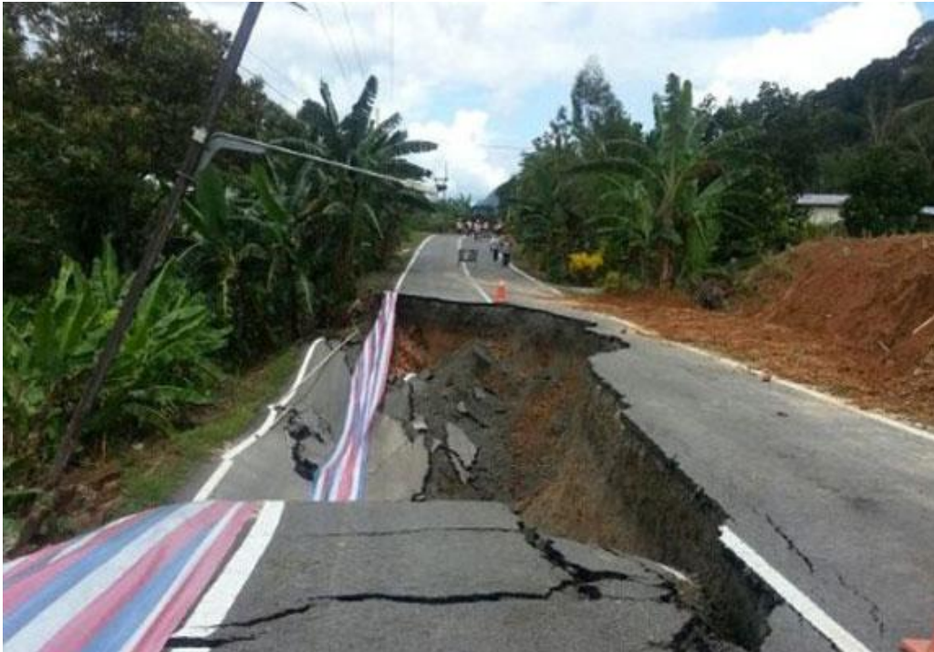
Figure 2: Road embankment failure ( https://adda.com.my/project-page/landslide-slope-and-road-embankment-failures-in-general/ )
