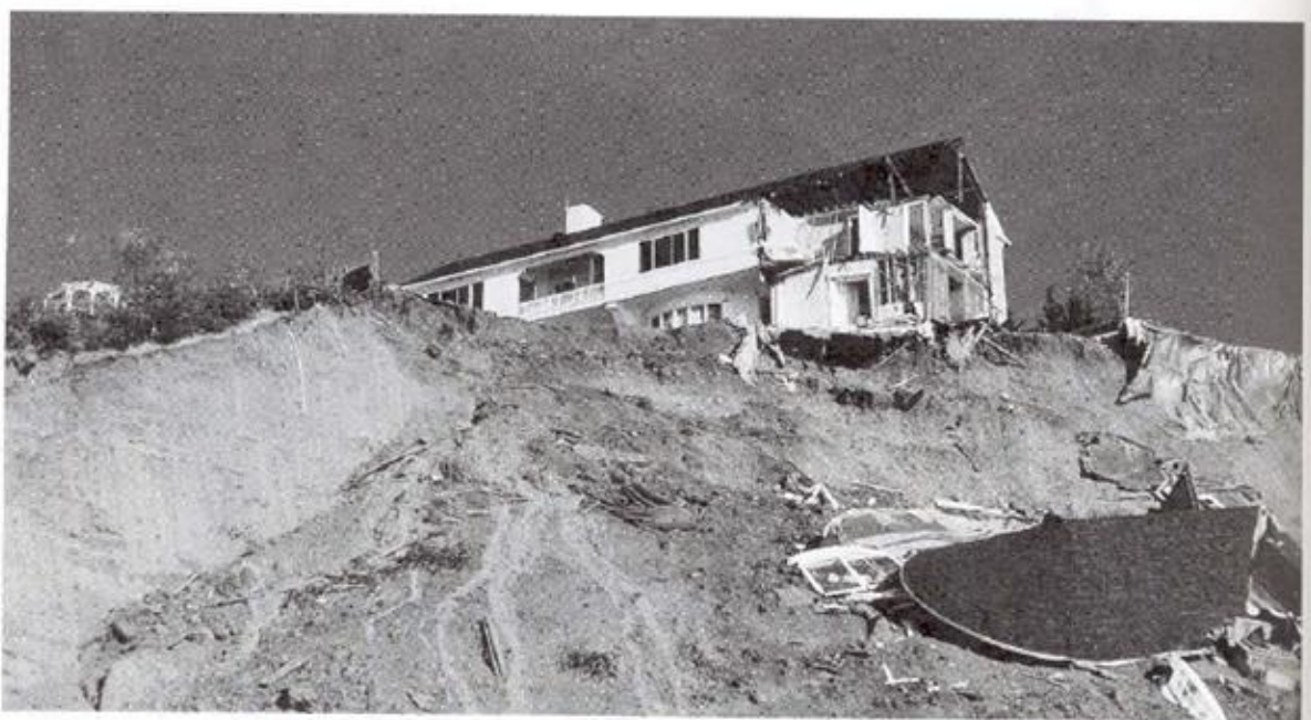
Figure 1: Collapse of a house caused by slope shear failure (Leverett Bradley/Tony Stone Images/New York, Inc., Budhu, 2015)
