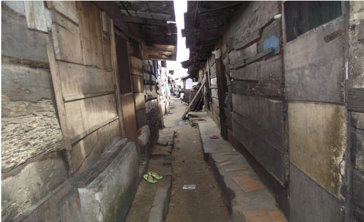
Plate 2: Deteriorated Buildings at Afikpo Water Front. (Source: Author’s Field Survey)
