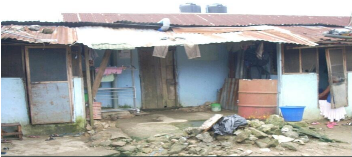
Plate 1: A Poorly Maintained Building at Afikpo Water Front. (Source: Author's Field Survey)
