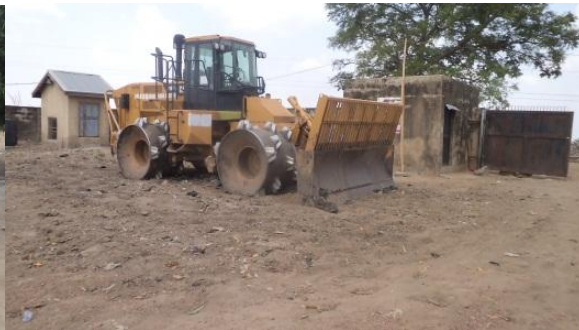
Plate 5: Land fill Compactor
