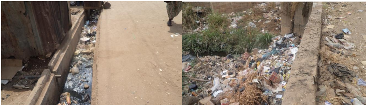
Plate 10: Poorly maintained gutter & drainage Plate 11: Blocked stream with waste, Karu Old Karu
