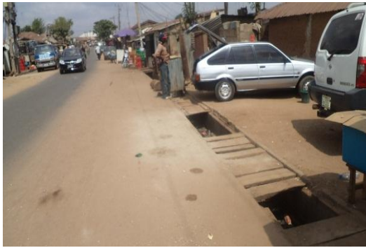
Plate 8: Clean gutters at Old Karu
