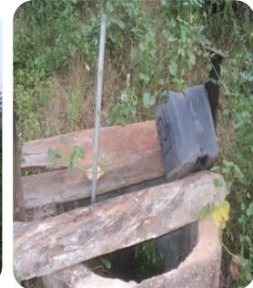
Plate 4: Poor aesthetic of the hand dug well in Uromi. Flood water carrying pollutants can flow into the well to pollute groundwater
