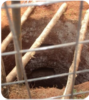
Plate 1: Hand dug well under construction in Uromi. The wells are locally dug to depths of 135meters to 150meters, shallow aquifers which are susceptible to pollutants.
