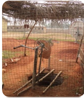
Plate 2: Hand dug well near completion in Uromi.
