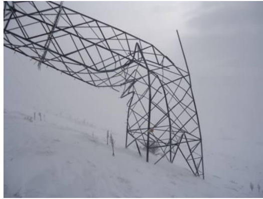
Figure 2: The bended transmission line tower
