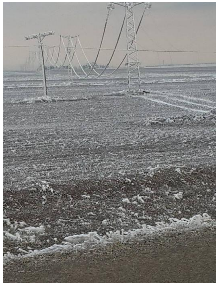
Figure 1: Pole of overturned distribution line in Turkey
