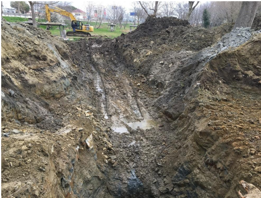
Figure 8: An image of the excavation in the study area
