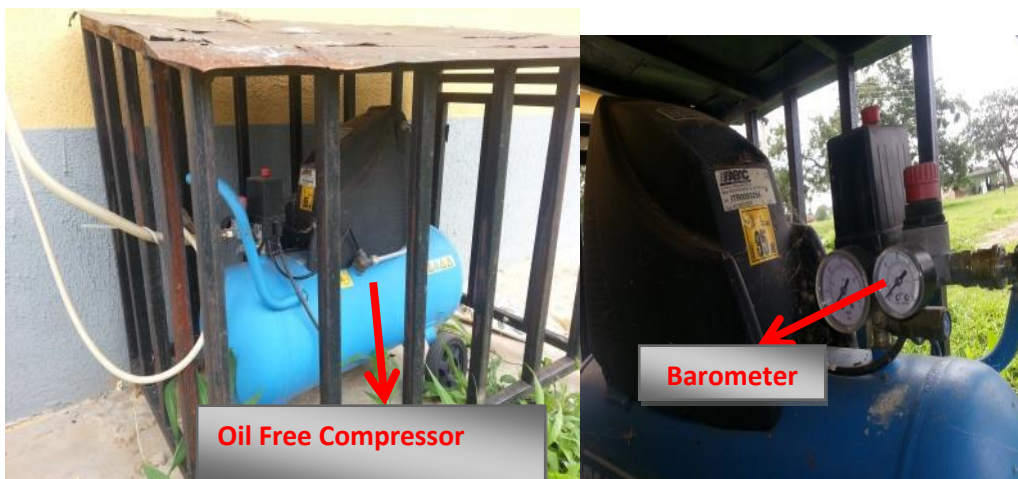
Plate 3: Oil- Free Compressor secured outside of the laboratory
