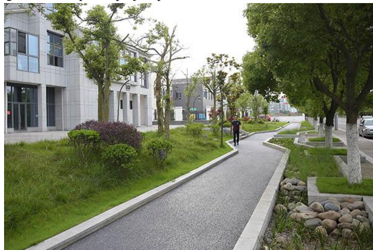
Figure 2: Pedestrian walk in Suining City Hedong New Area on a permeable green road
