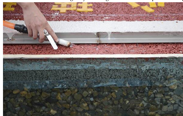
Figure 3: The staff in the Suining City Hedong New Area test gravel penetration of the water absorption effect
