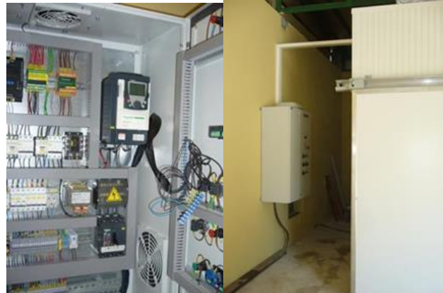
Figure 3: Electrical control box
