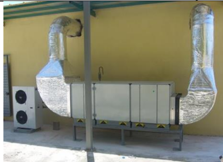
Figure 2: Air-conditioning unit, suction and pressure channels
