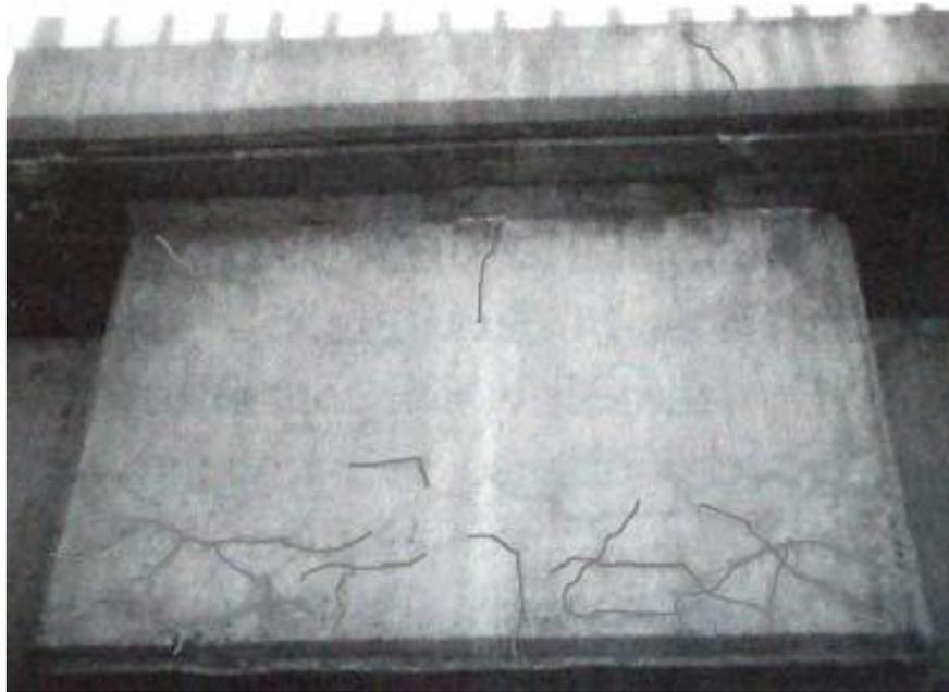
Figure 2: ASR impact on concrete
