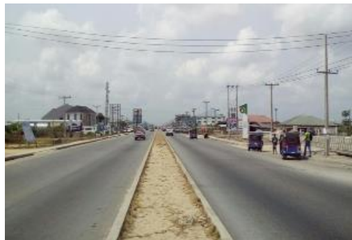
Plate 4: Isaac Adaka Boro Road one of the Major Road in the Study Area without Drainage Source: Researcher's Fieldwork, 2016
