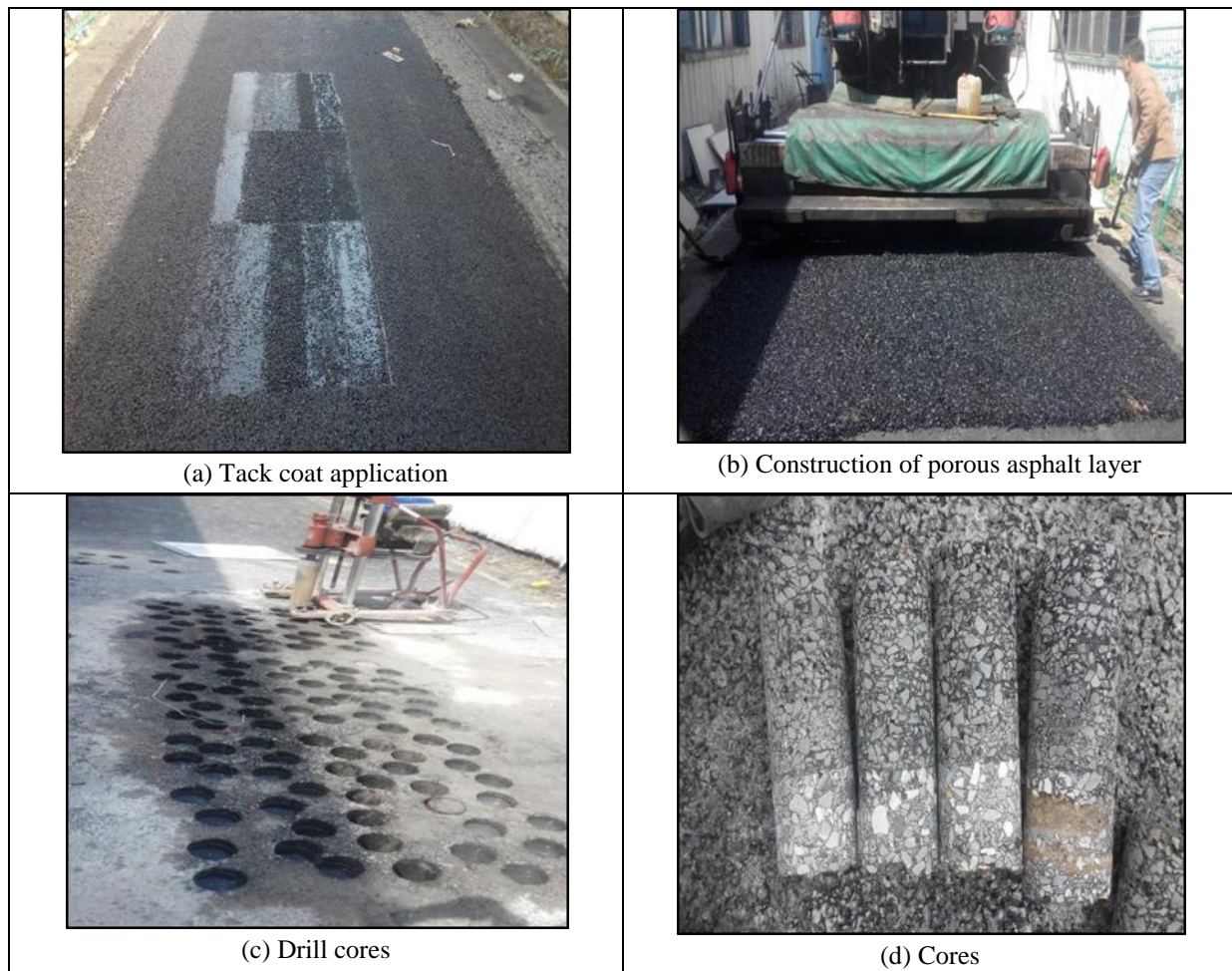
Figure 9: Construction of test road
